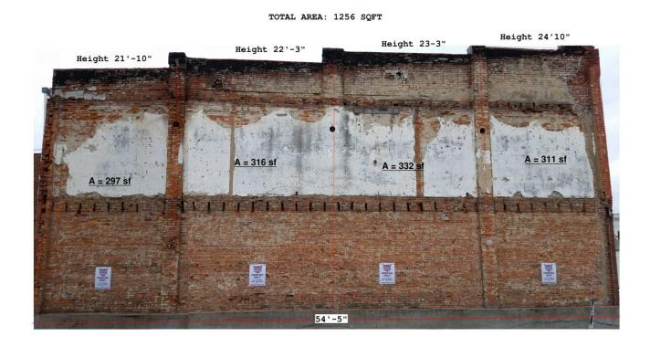
The building side will be prepped with an EFIS (Stucco) finish which will provide a solid color and surface for the mural. The base color can be white, other color options are available.
